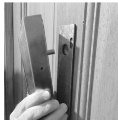
3. With door open, insert key safe
